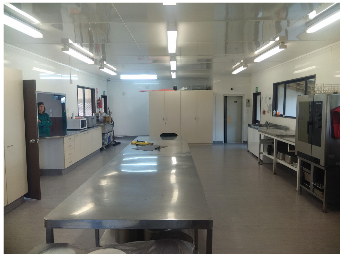
Existing Kitchen showing end Wall where Bathroom Rebuild Joins
