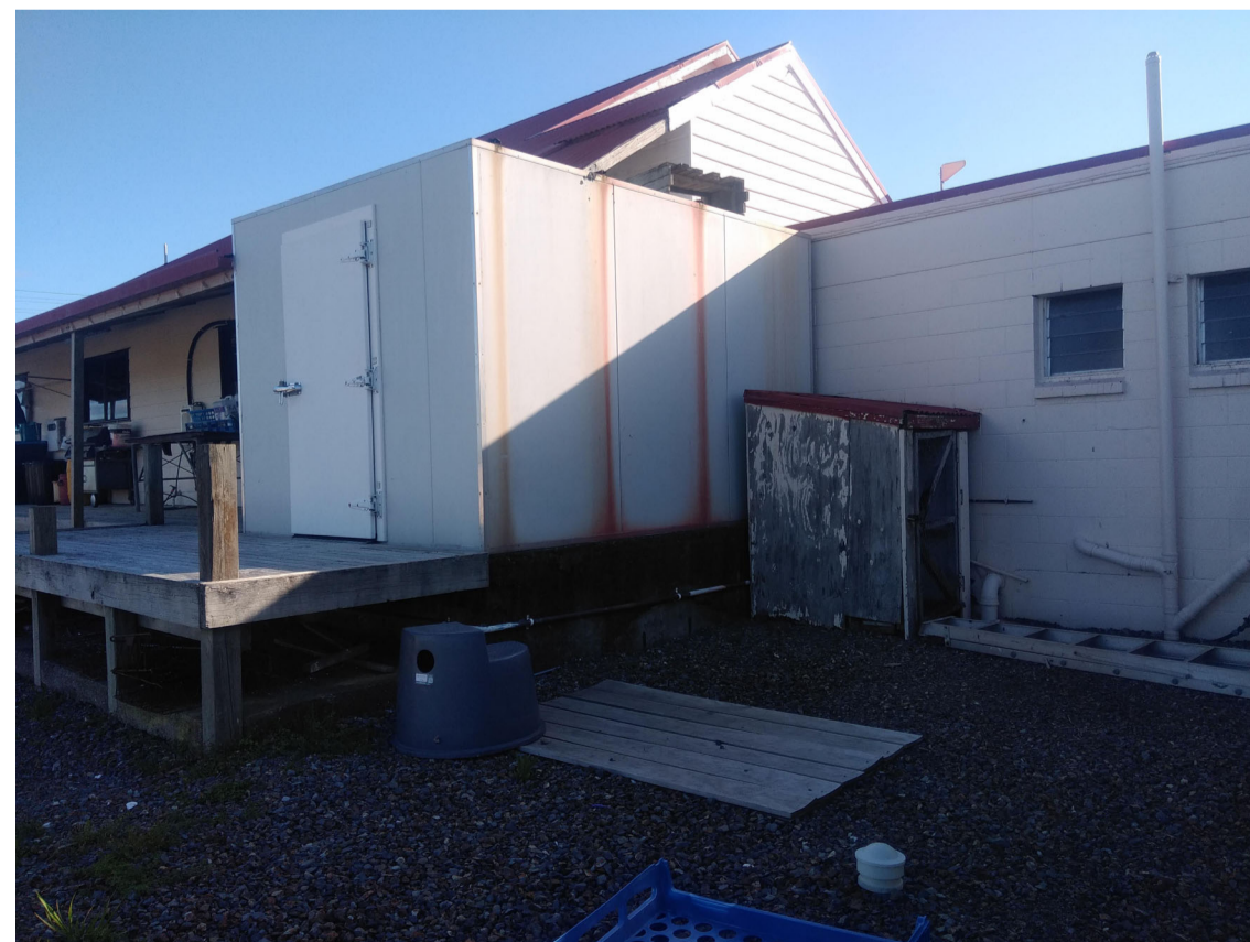
Existing Chiller - New Roof partially covers the Chiller Room
