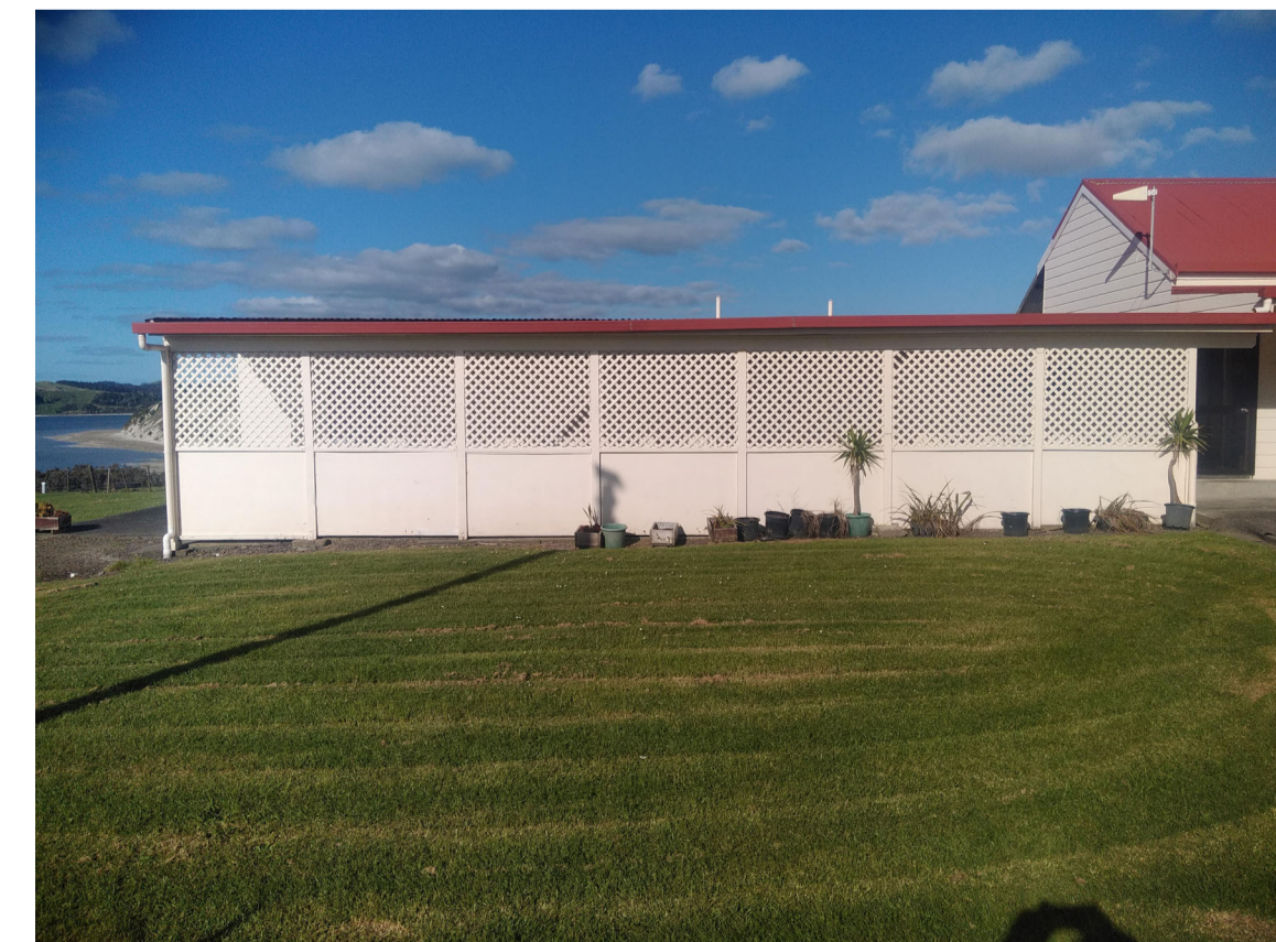
Existing Screened Walkway beside Toilet Block To be Demolished
