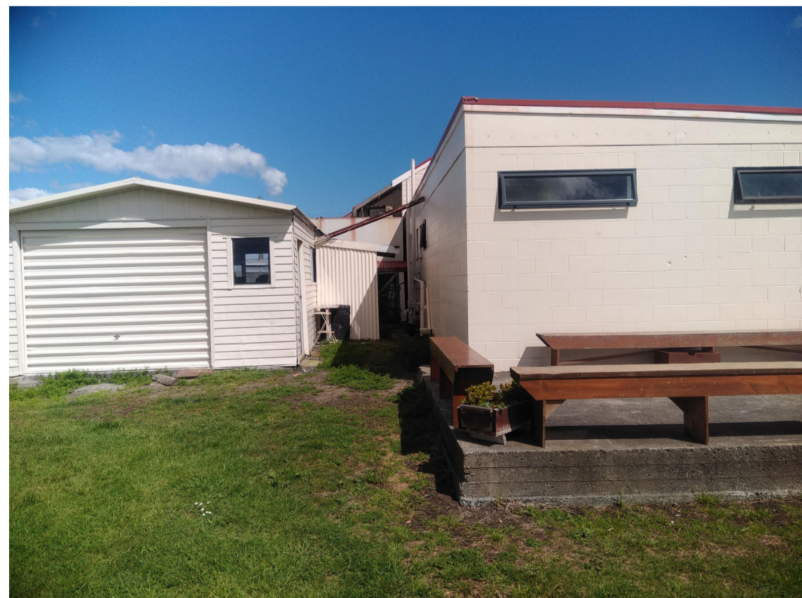
Shed and End of Existing Bathroom Block All to be Demolished
